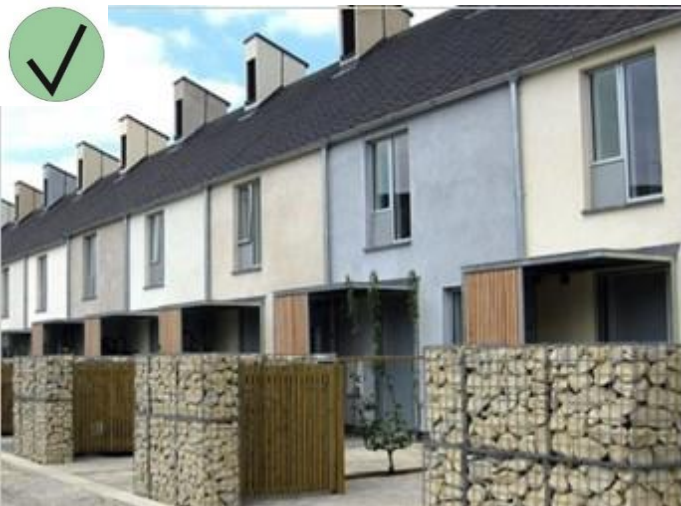
Left middle: Bin storage at the front of properties is well integrated into the scheme and frontage space design, defining the boundary between the street and house frontages in a visually unobtrusive way.
