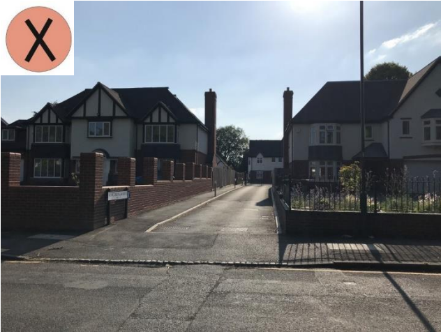
Figure 2.1 (left top): tarmacadam drive into site, enclosed by walls and timber fencing:
