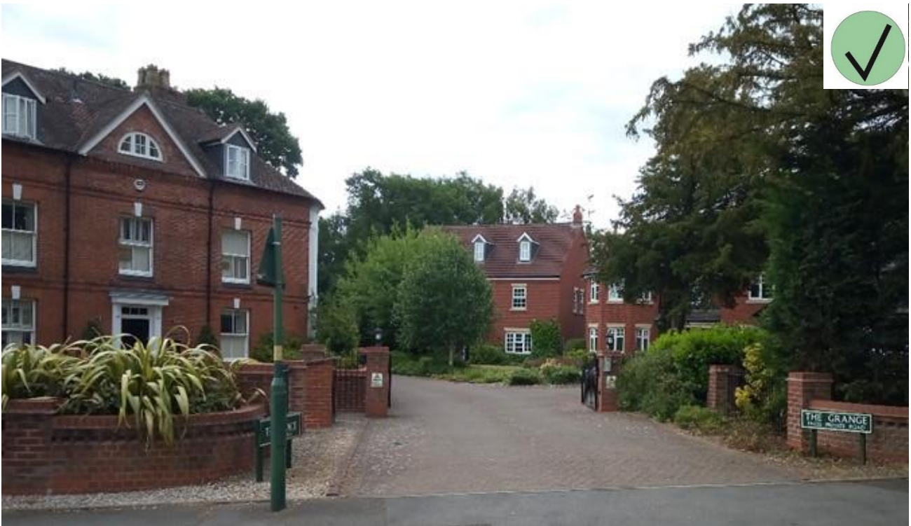
Figure 12.1 (above): The scale and appearance of this new access into a backland development is sympathetic to its context. The entrance is well marked, but not over-engineered or unnecessarily wide. Rather than using prominent highway kerbs and tarmacadam, the driveway and edging materials create a pedestrian character for both entrance and driveway. The continuous, flush footway along the frontage signals to drivers a need to give way to pedestrians when entering or exiting. The entrance design makes clear that this is a secondary, or ‘subservient’ side street off the main frontage street. The backland buildings are visibly located and face out onto the main frontage, resulting in a positive connection with the existing street and neighbourhood.
