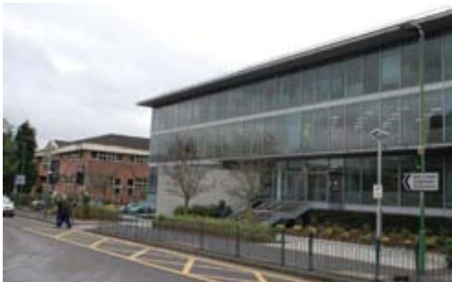
Commercial buildings along Homer Road
