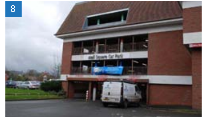
8 Frontage along Warwick Road: Photo shows both multi- storey and ground level car parking along Warwick Road. This creates a poor frontage to Warwick Road and a negative pedestrian experience.
