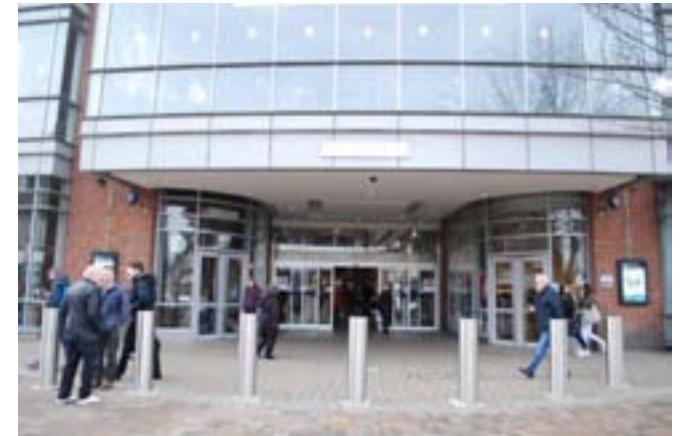
Entrance of Touchwood Shopping Centre
