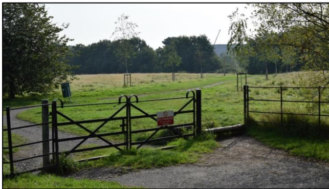
7. The site looking east from former carriage drive east of The Grange, JLR logistics centre under construction to right of centre
