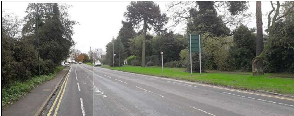
3. View from site entrance south eastwards to The Green (not visible), The Laurels to right
