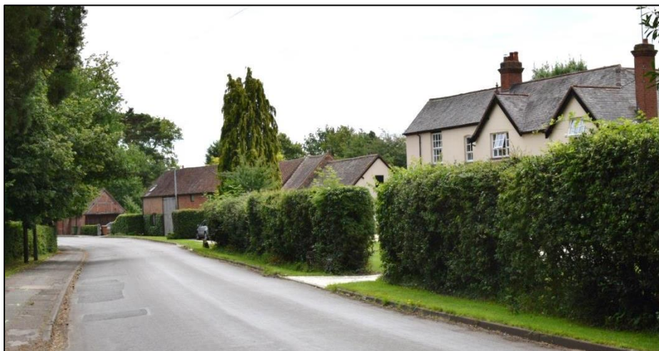
7. Grove Farmhouse and barns to left, looking east on Grove Road
