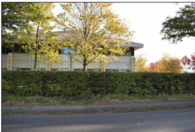
3. Typical building at the south edge of TRW site
