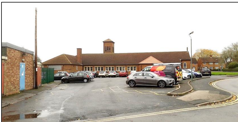
3. South face of church hall showing opportunity for enhancement of setting
