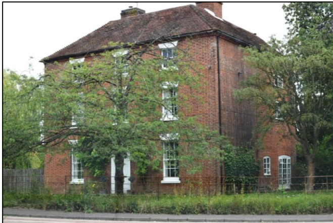
1. Rotton Row Farmhouse from Grove Road
