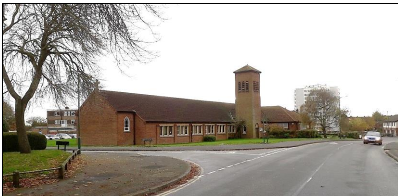
2. North end of church showing open space and higher ground contributions to its setting and focal value of tower as a feature
