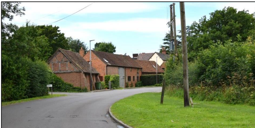
6. Grove Farm east and west barns looking west on Grove Road with site opposite
