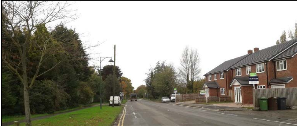
1. The site beyond new build houses on right looking north west on Birmingham Road
