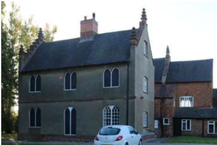
Figure 13 Park Farmhouse, north elevation
