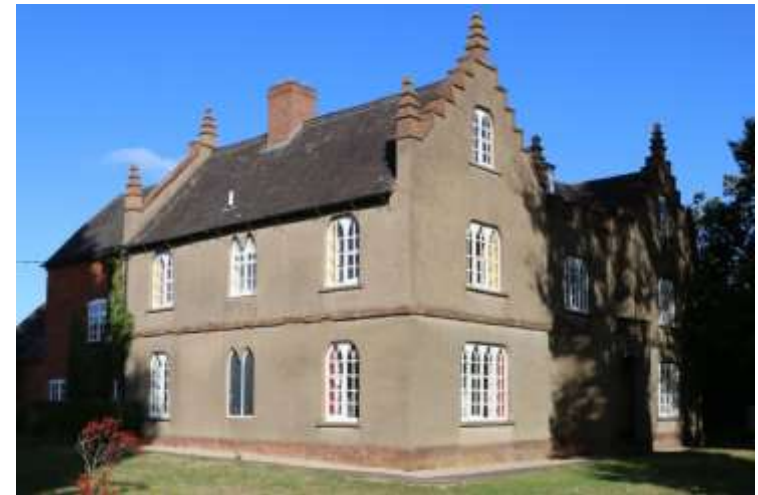
Figure 14 Park Farmhouse, east elevation facing Packington Park
