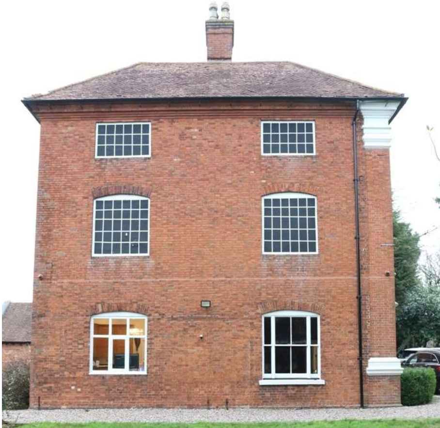
Figure 14 Light Hall; east side elevation
