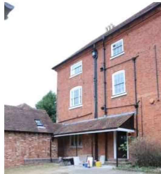
Figure 13 Light Hall; south rear elevation
