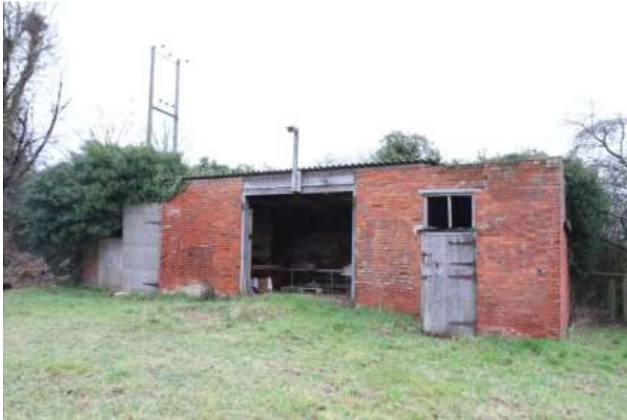
Figure 16 Light Hall; outbuilding adjacent to former walled garden
