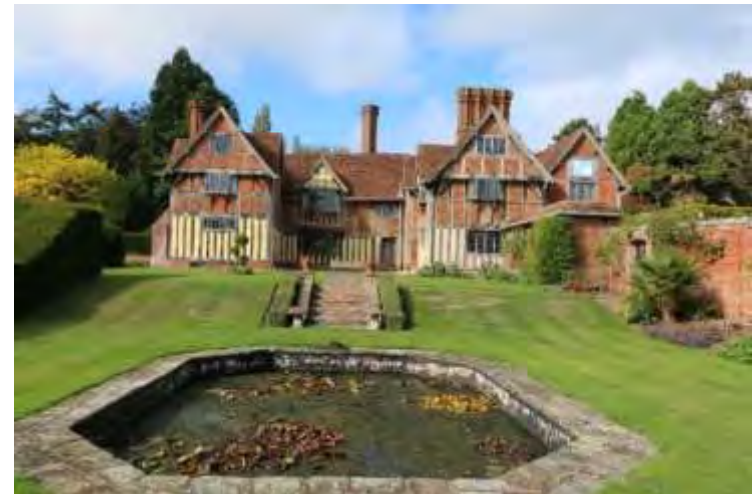
Figure 12 Grimshaw Hall; east rear elevation
