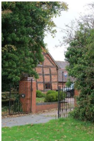
Figure 11 Gable end of Whitlocks End Farm; Listed Grade II
