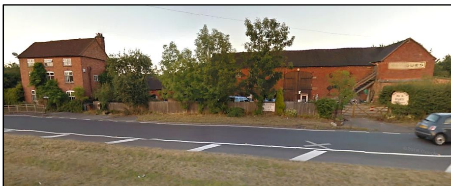
10. Skew Bridge Farm with imposing 19 th century threshing barn and outbuildings, to opposite side of A452 (Google Streetview image)
