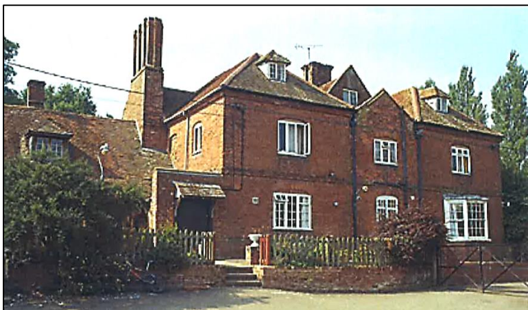
13. North façade to farm courtyard (image from HS2 website)
