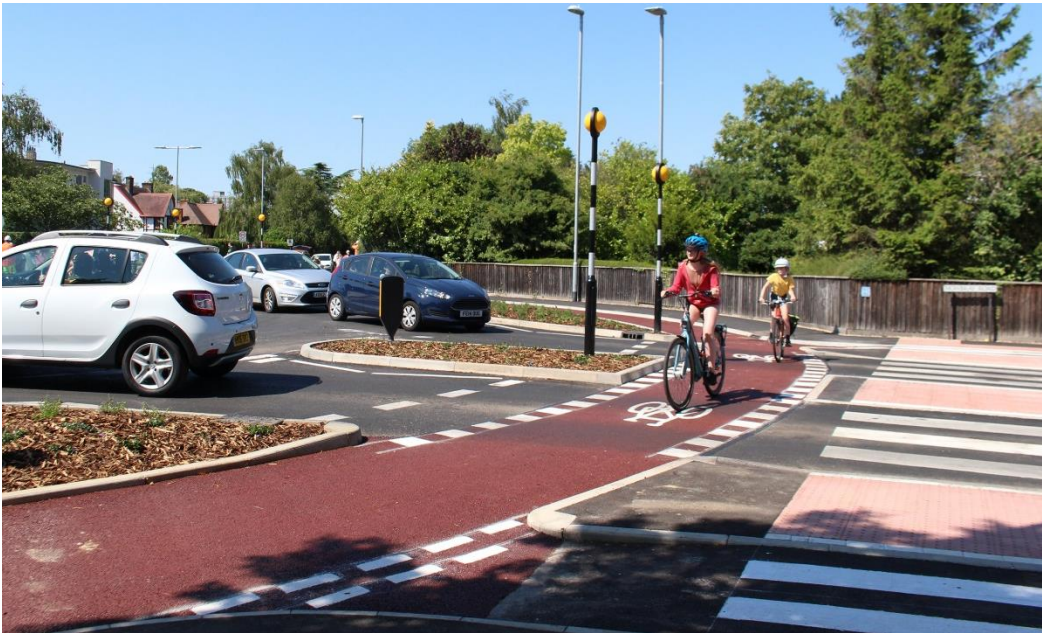
Figure 4.12: Fendon Road Roundabout in Cambridge
